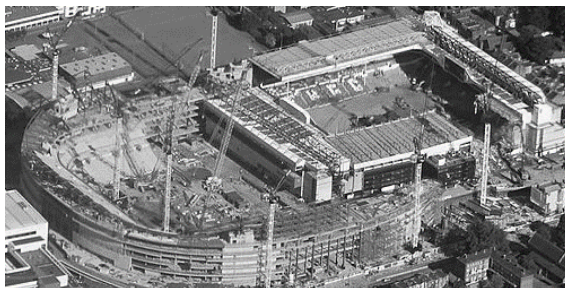
Dicestraat in May 2010 with new stadium being built next to it. West Stand partially demolished.
