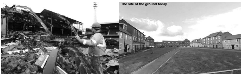
The Forum demolition and the grounds today
