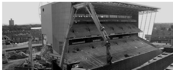
The demolition of Nodir Stadium
