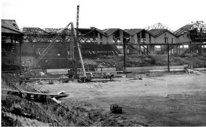
Construction works at Ostric Grounds in 1945
